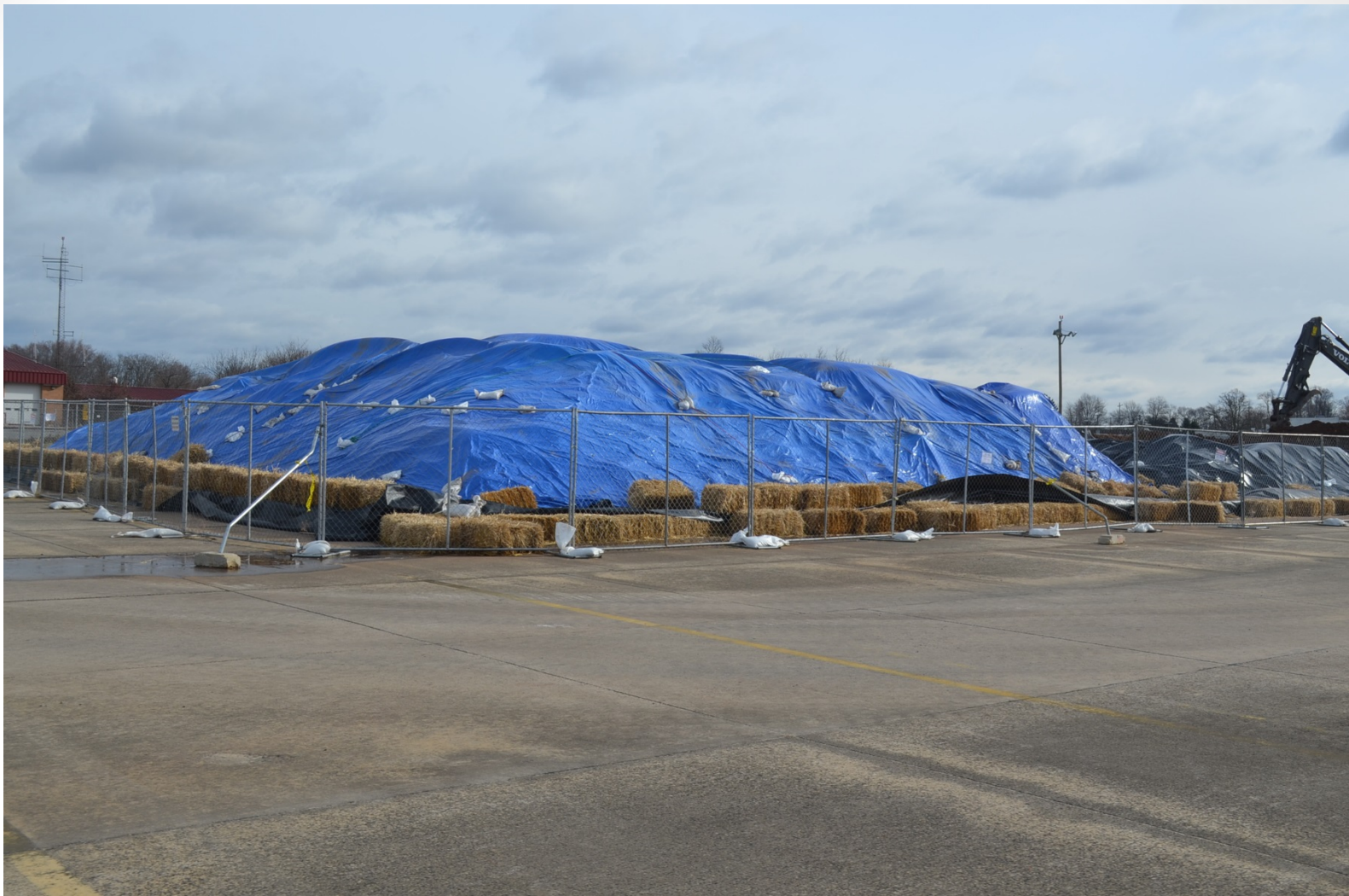
Navy Soil Removal Project – NAS-JRB Willow Grove Photo taken 11-28-2018
